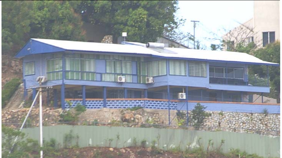
THIS photograph shows the guest house on Paga Hill in Port Moresby, National Capital District.
