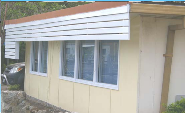
The newly renovated transit facility for seafarers and PNGPCL stakeholders in POM.
